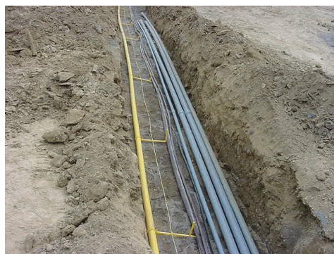
buried in the ground
